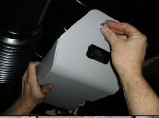
3. Lift canister panel into position and secure using M8 x 25 bolts, spring washers and flat washers.
